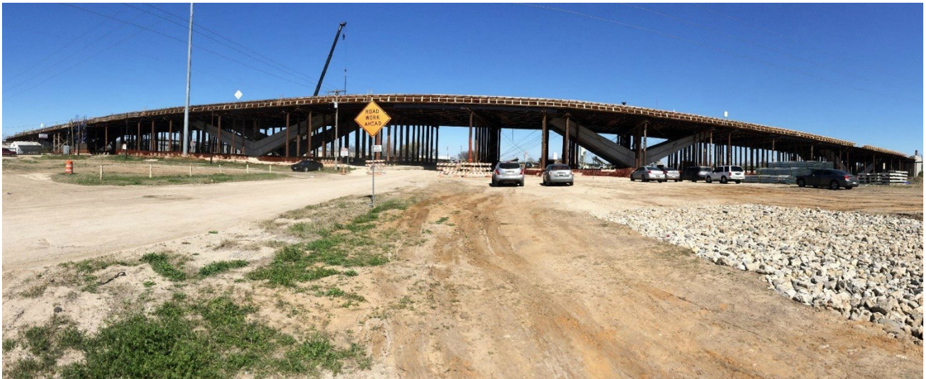
(White Settlement V-Piers for bridges under construction)
