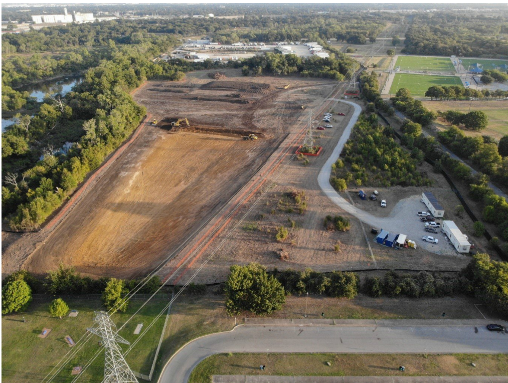
(Construction progress at Gateway Park Site H)
