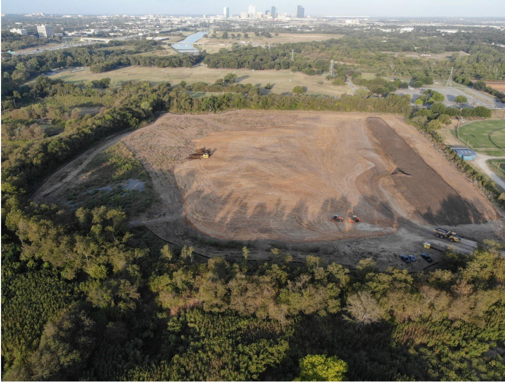
(Construction progress at Gateway Park Site I)
