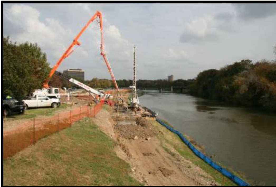
(Construction for Trail Improvements at Rogers Road and University Dr.)
