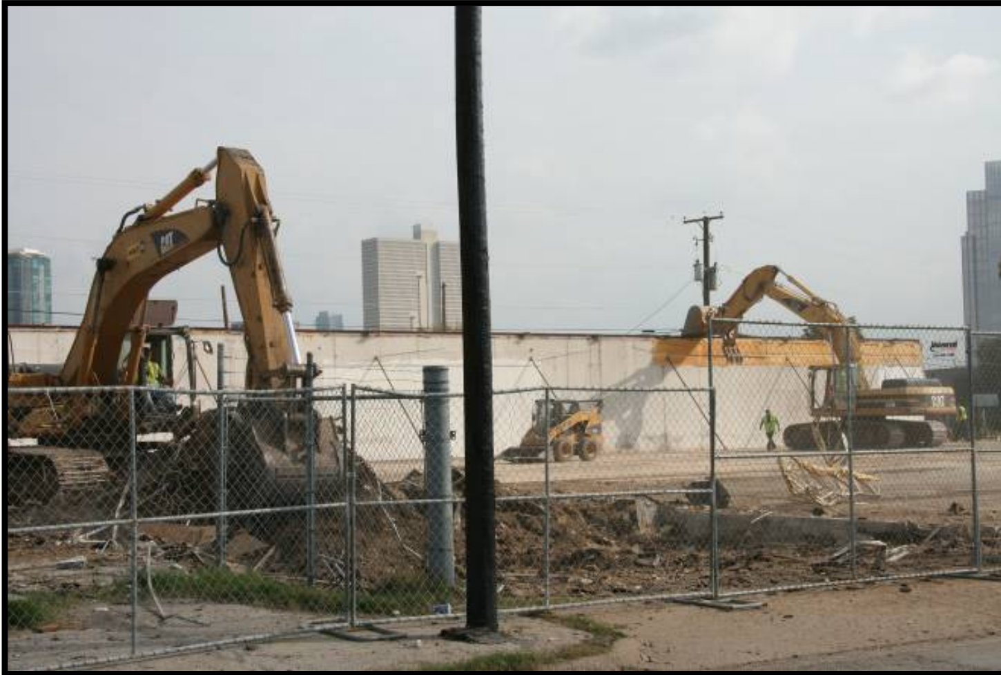
(Demolition work being done off White Settlement and Greenleaf)
