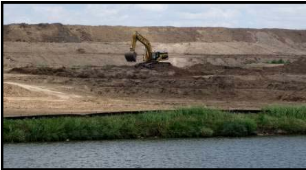
(Construction of Valley Storage off Northside Dr.)
