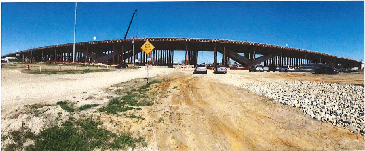
(White Settlement V-Piers for bridges under construction)
