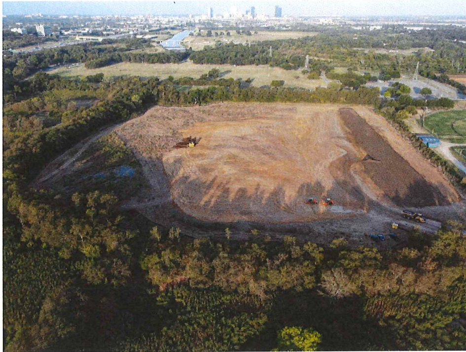
(Construction progress at Gateway Park Site I)
