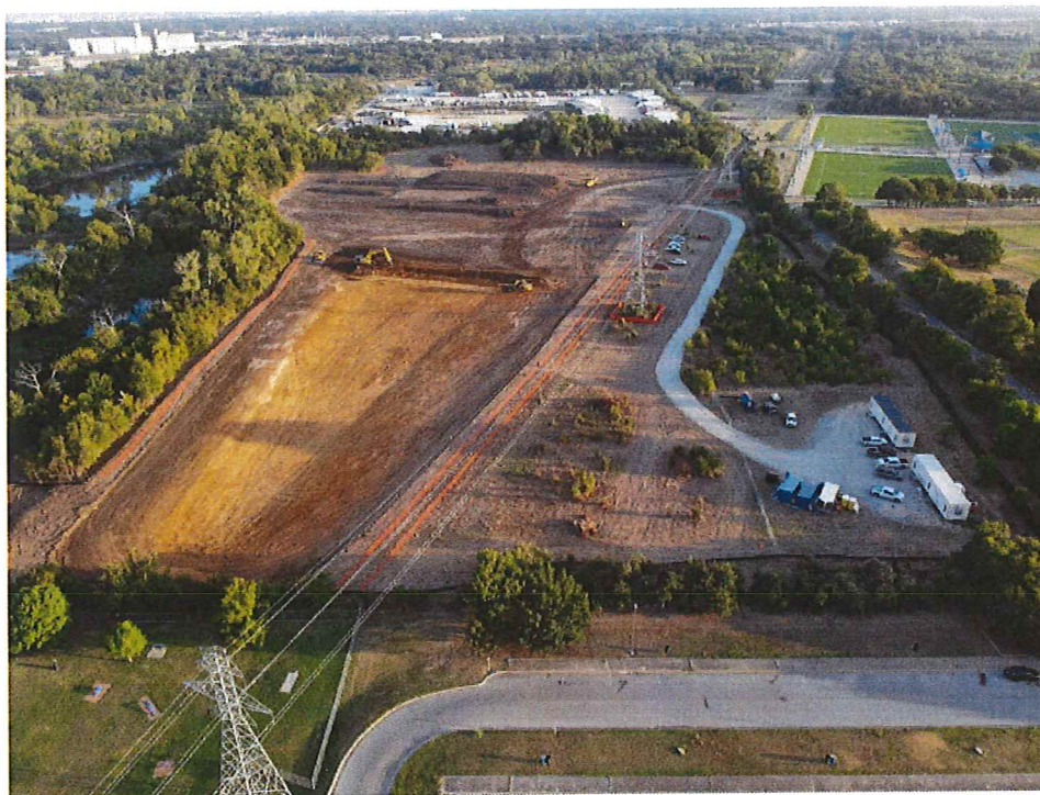
(Construction progress at Gateway Park Site H)
