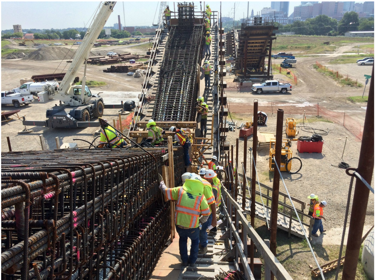
(White Settlement bridge construction)
