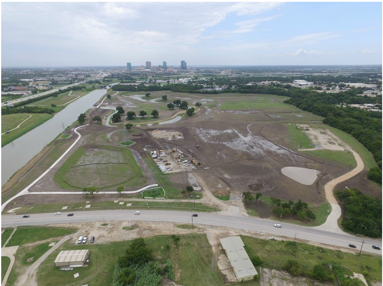
(Excavation work at Gateway Park)
